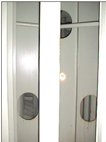
Figure 13: Existing Stability Tank Central Partition and Openings
